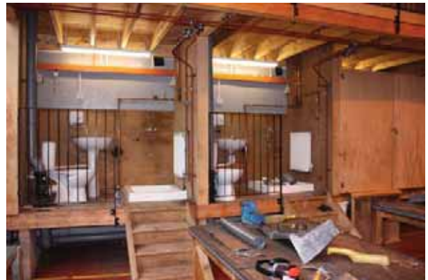
Plumbing workshop Forth Valley College (photo: AMA)
